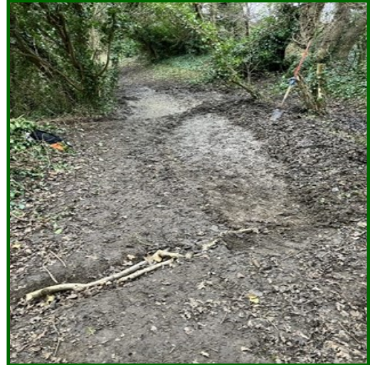
Path below Conger Hill with free-flowing spring. Mulch has been scraped away to provide a gravelly surface
